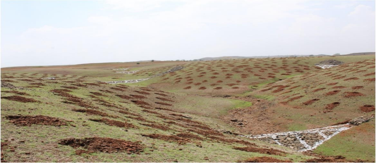
(Integrated watershed structures in Mohaliya Village, Barwani, Madhya Pradesh)
