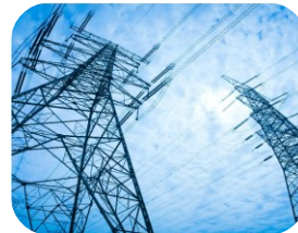
Traditional Overhead conductor
