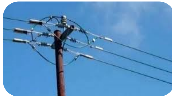
Covered conductor ( 20 km – 60 km from coast)
