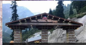
Atal Tunnel, India
