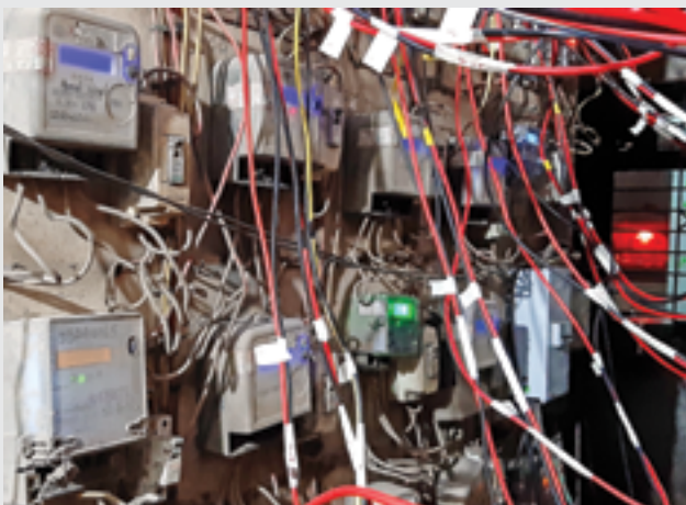
Meter replacement at Bhiwandi
