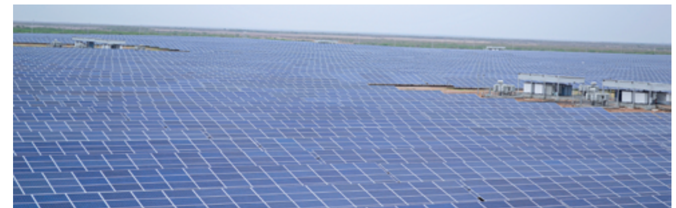
Charanka Solar Plant
