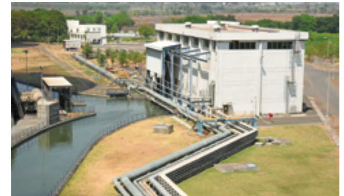
Efficiently utilizing water for cooling at SUGEN
