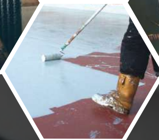
Road Surface Treatment
