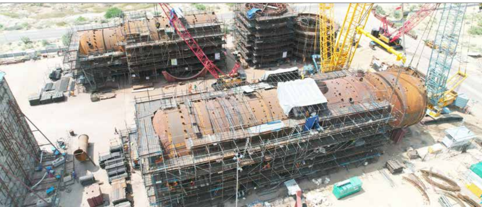
FCCU Package being manufactured onsite at Refinery in Barmer, Rajasthan
