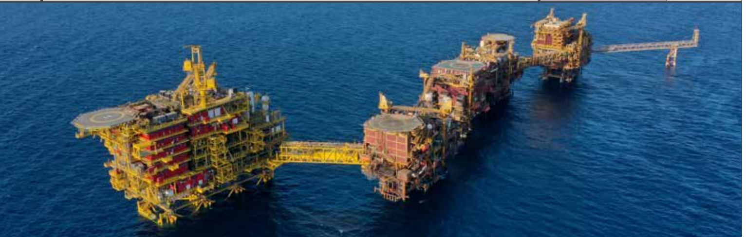
New Water Injection System - R Project for Oil & Natural Gas Corporation
