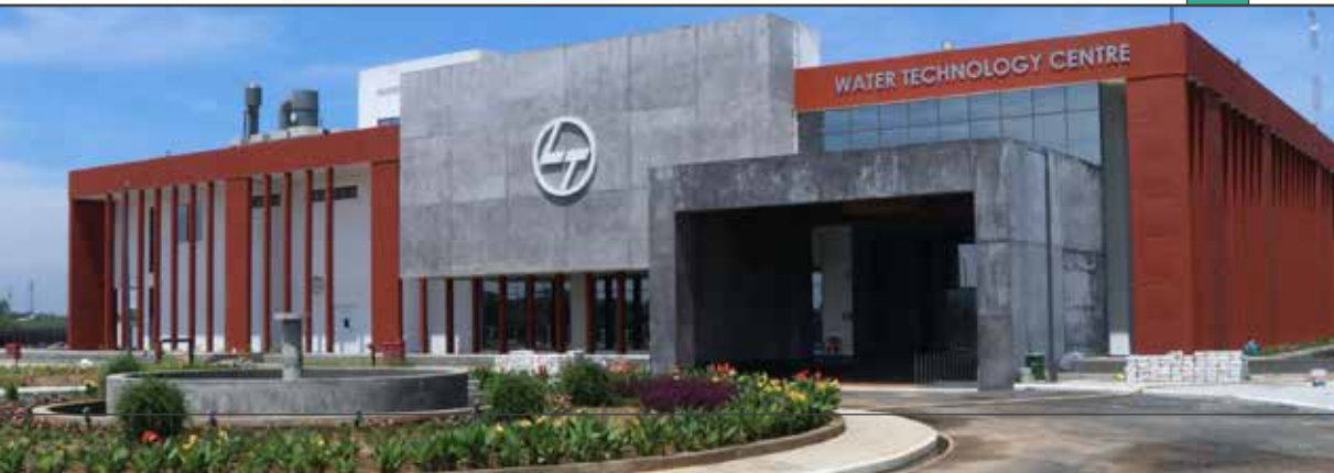
Water Technology Centre, Kancheepuram
