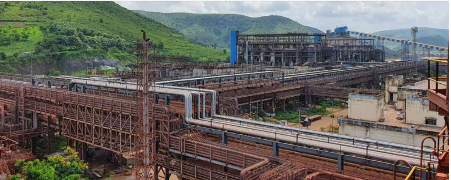
Utkal Alumina Expansion Project, Rayagada, Odisha
