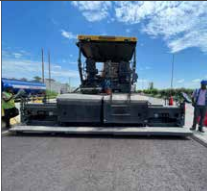
CCPR implementation at Meerut-Aligarh-Ghaziabad road project
