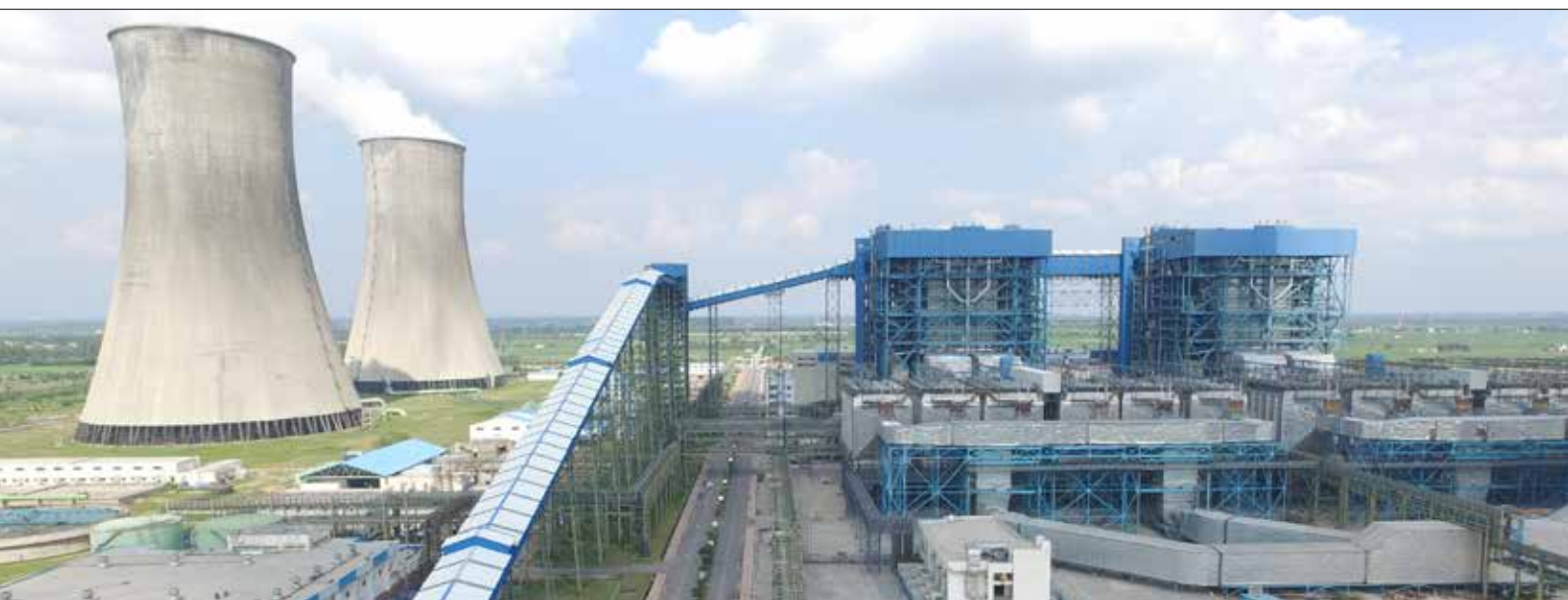
2x700 MW Supercritical Thermal Power Plant, Rajpura, Punjab
