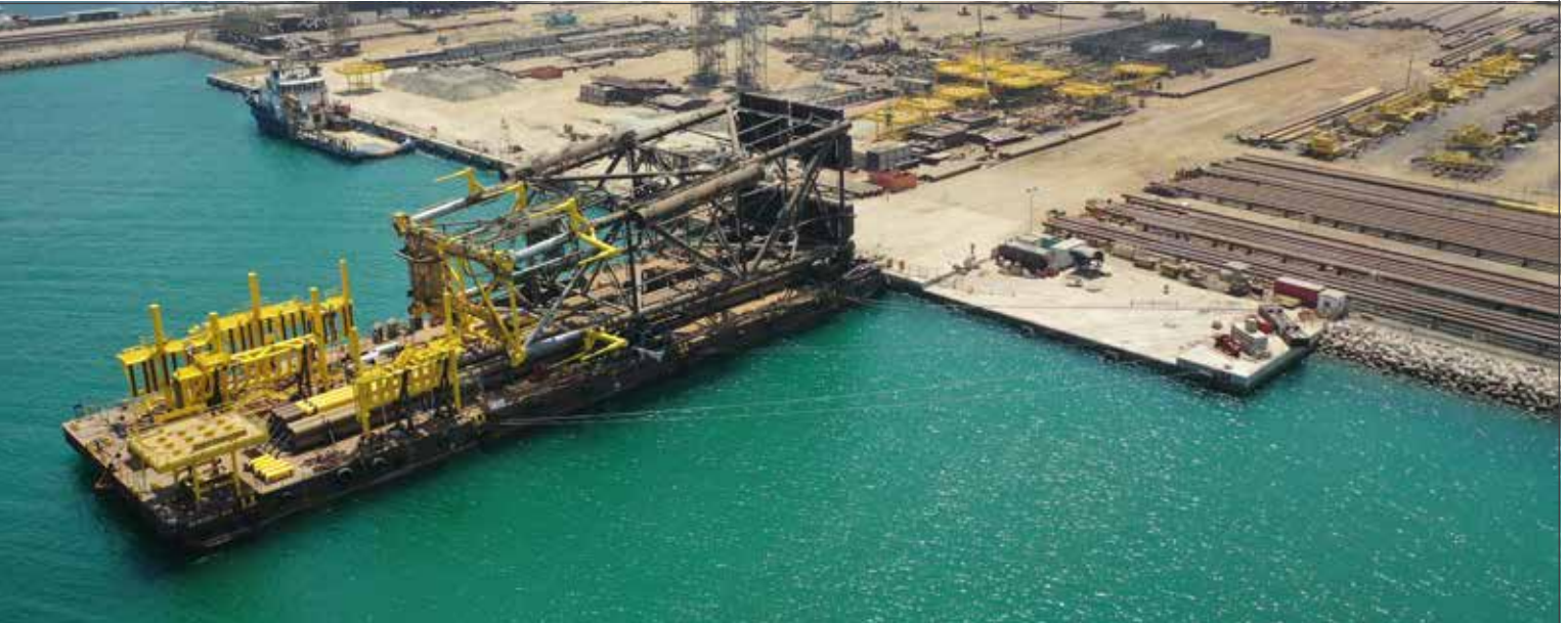
One of 28 Jackets being shipped to Zuluf Field, Saudi Arabia
