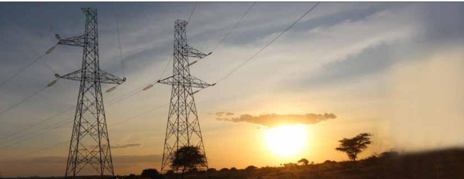
SGR 2.2 Transmission Line, Tanzania
