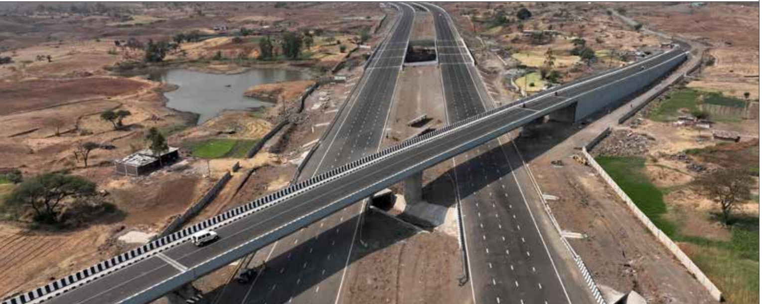
Madhya Pradesh Expressway project, part of the Delhi-Vadodara Expressway project
