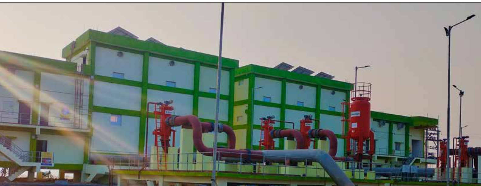
Mega Lift Irrigation Project Cluster IV, Odisha
