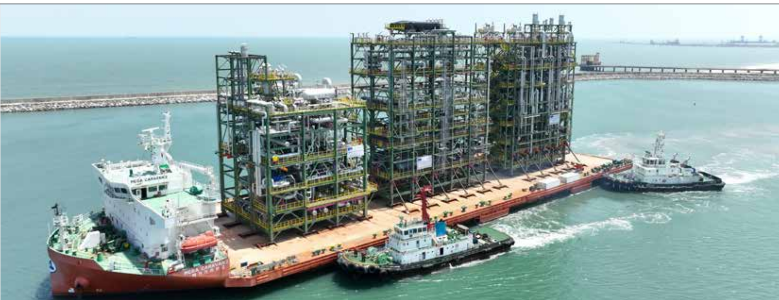
Sailaway of Process & Piperack Modules from MFF Kattupalli for Gasification Plant for Linde, Singapore
