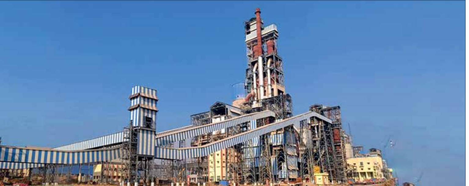
RAMCO Cement Plant, Kurnool, Andhra Pradesh
