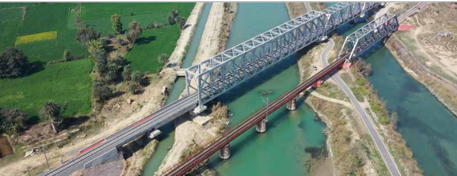
Khurja-Khatuali section of Eastern Dedicated Freight Corridor
