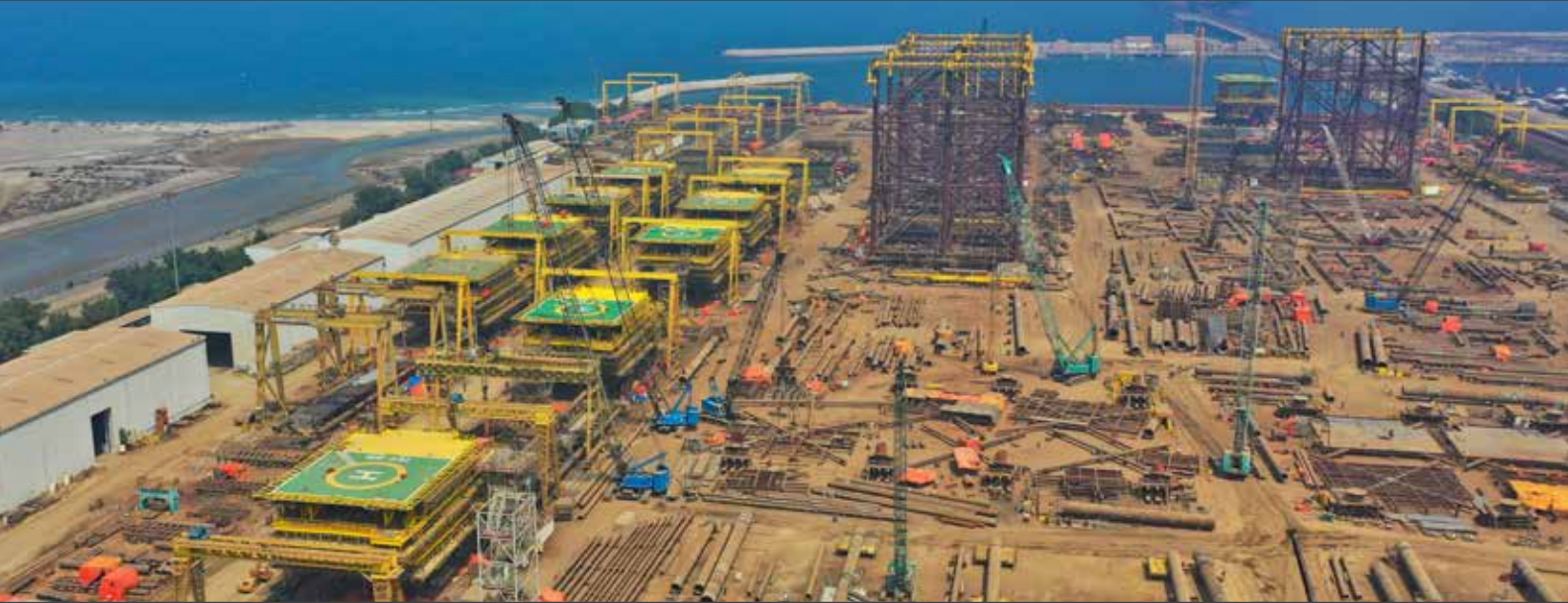
Offshore platforms being fabricated at Sohar yard, Oman
