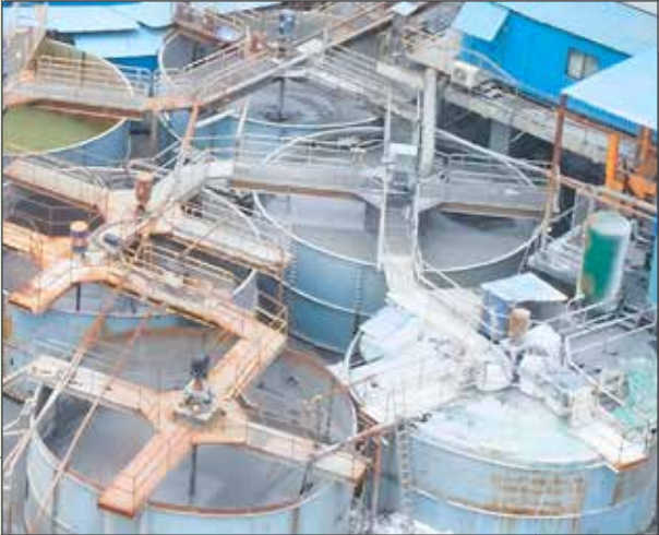
Tunnelling slurry processing at Mumbai Coastal Road project
