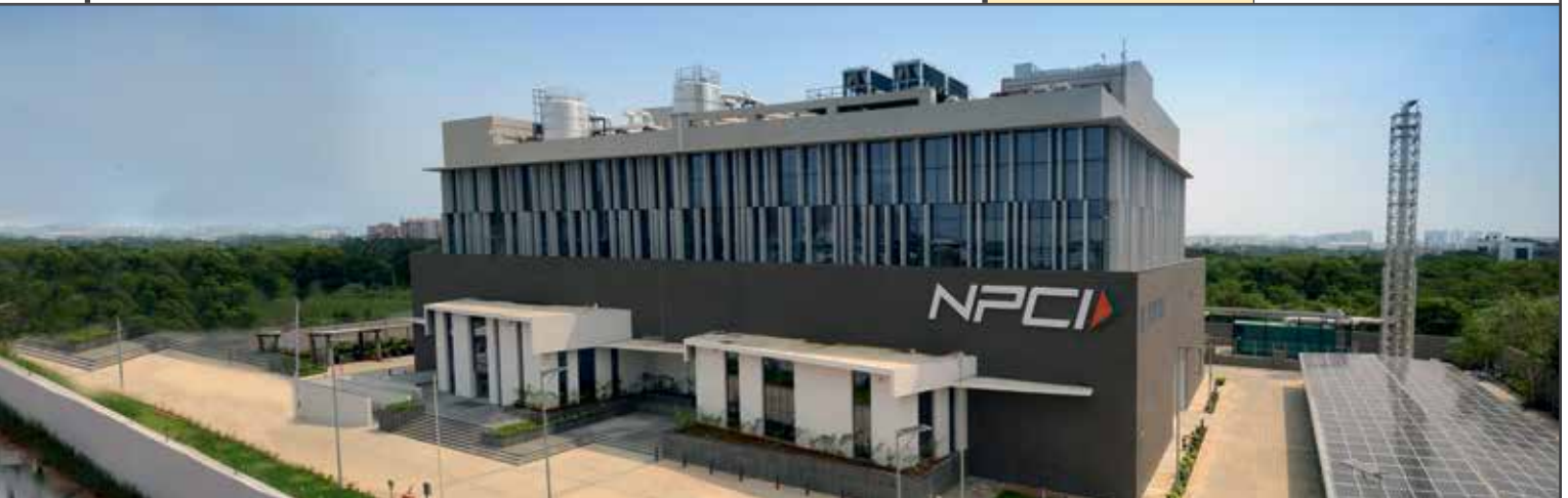
NPCI Data Center, Chennai
