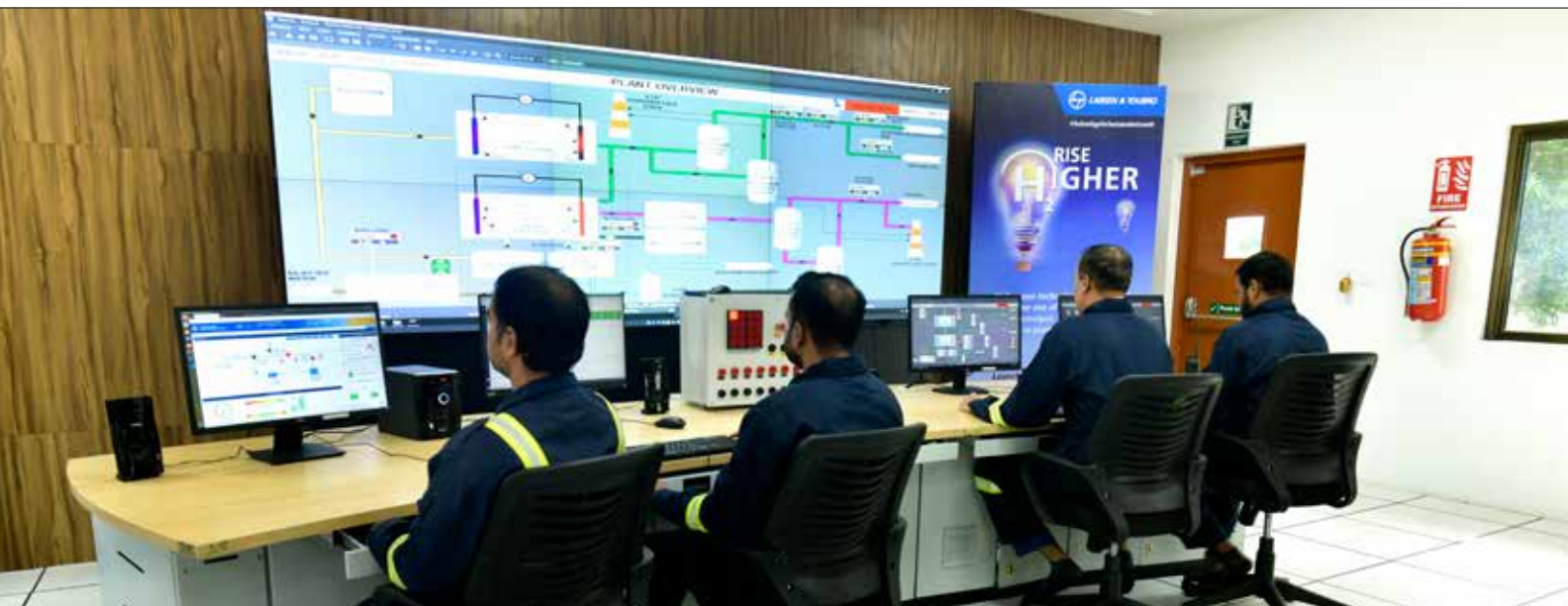
Control Room of the Green Hydrogen Plant in Hazira, Gujarat
