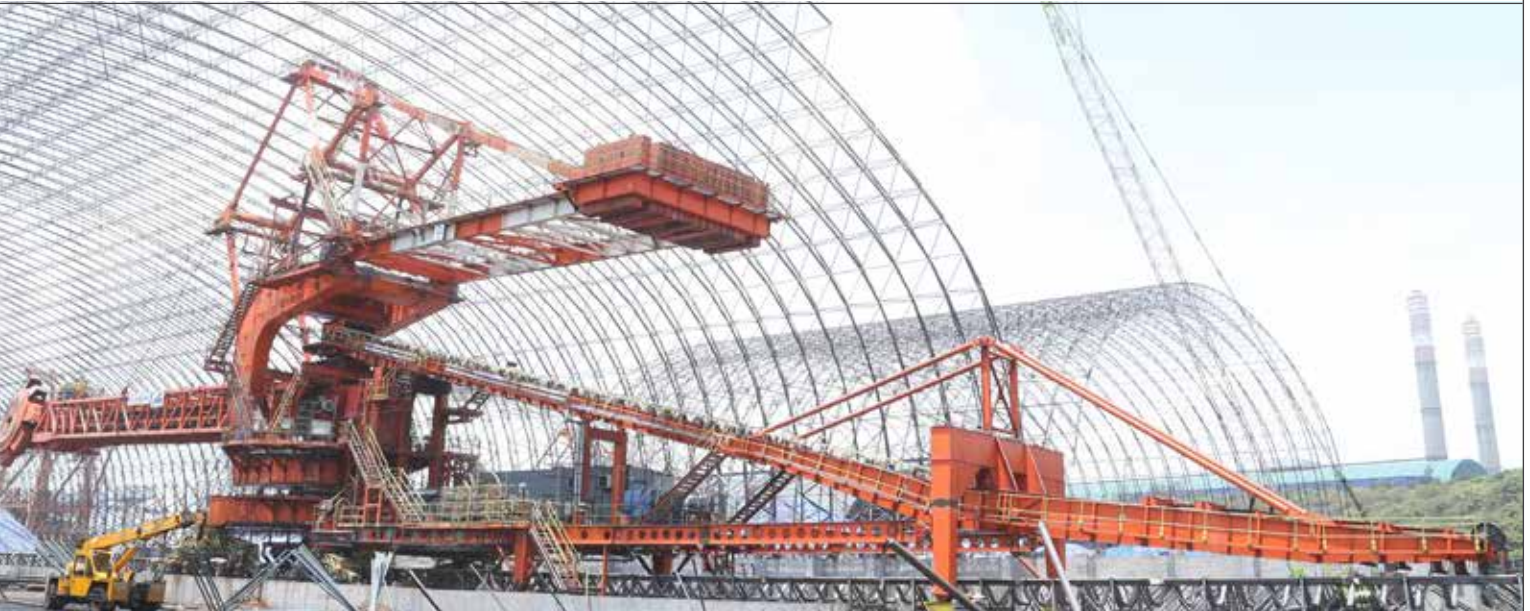
India's largest capacity Stacker-Reclaimer, JSW Jaigarh
