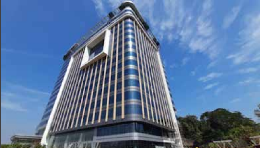
A.M. Naik Tower, Mumbai
