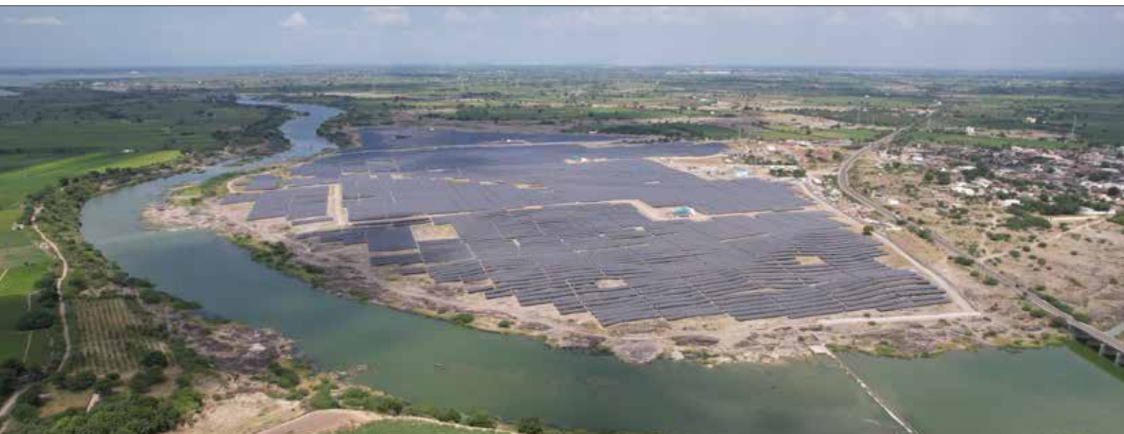
40 MW Solar PV Power Plant, Haripar, Gujarat
