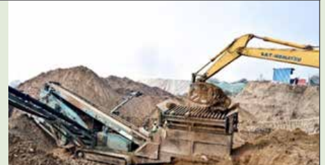
Reuse of excavated material at Delhi Airport project
