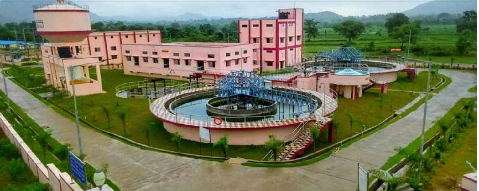
Nuapada Water Treatment Plant, Odisha
