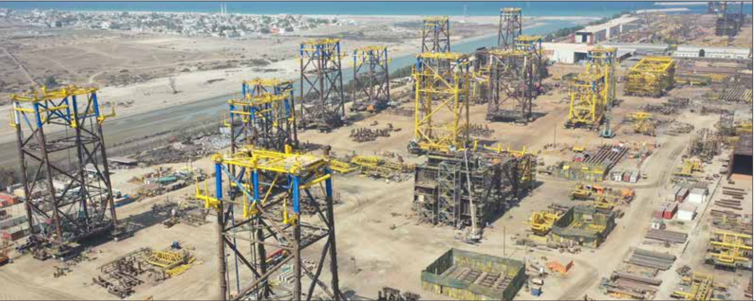
28 Jackets being fabricated for Zuluf Field, Saudi Arabia
