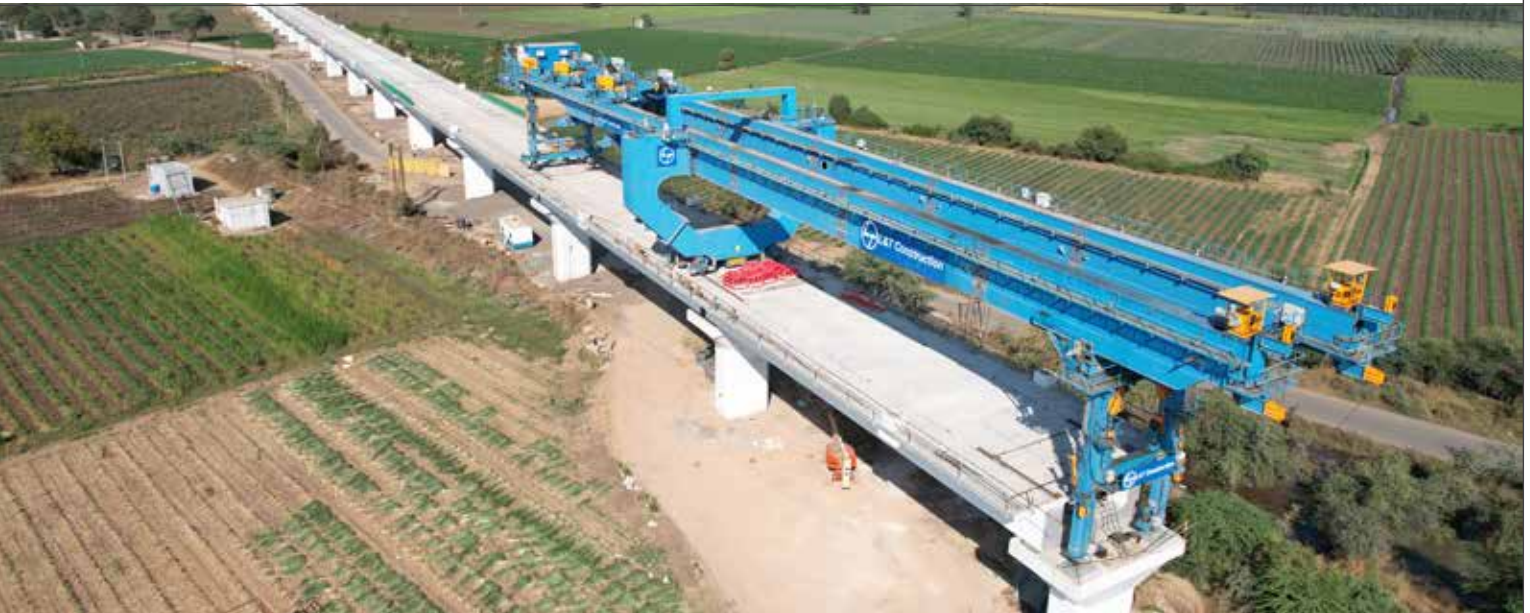
Mumbai-Ahmedabad High Speed Rail project
