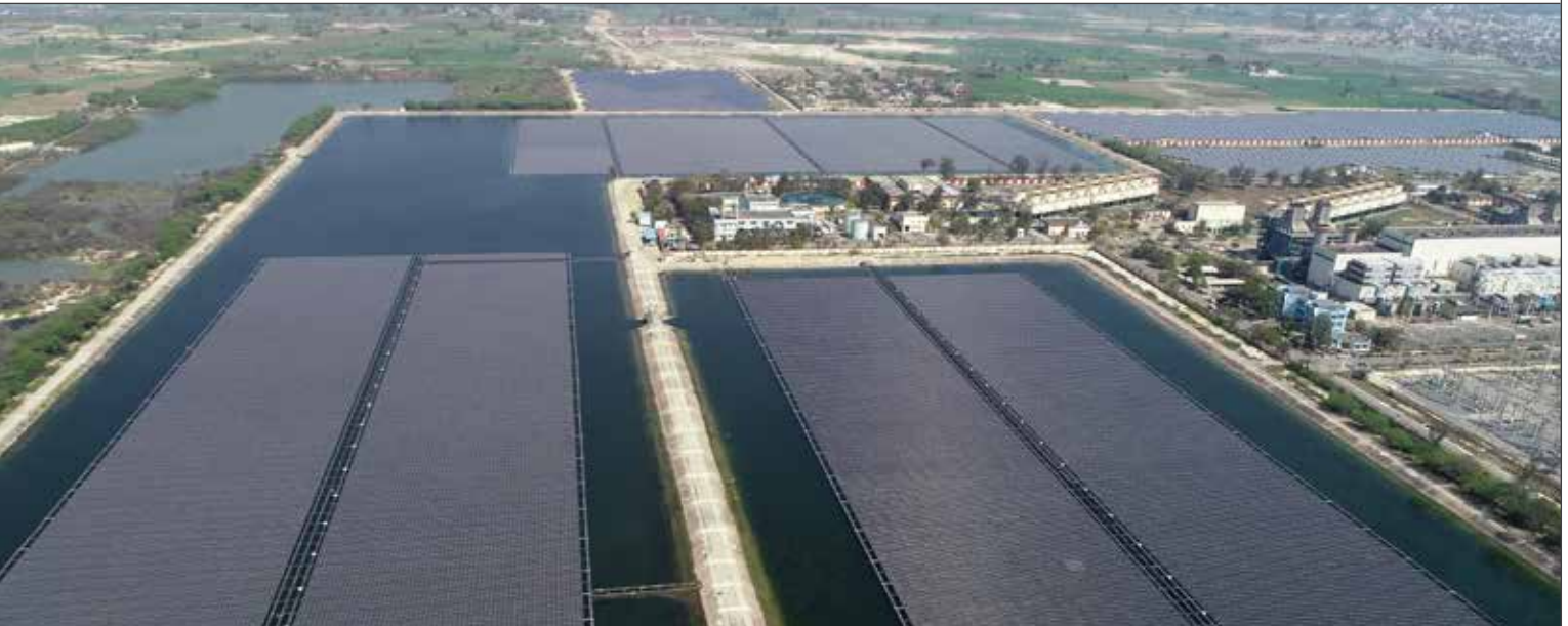
20 MW Floating Solar PV Power Plant, Auraiya, Uttar Pradesh
