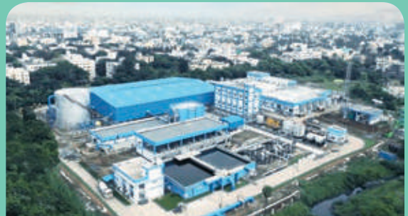
45 MLD Koyambedu TTRO Recycle Reuse Plant Chennai, India One of the largest and most technologically advanced water reuse plants in India ensuring Chennai's water security
