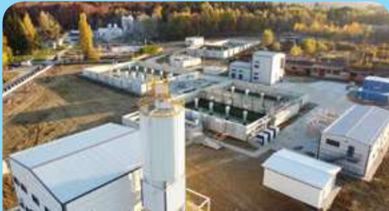
PUROLITE WWTP, Victoria, Romania A global reference for advanced industrial applications for WABAG, using high-end technologies to meet stringent discharge conditions.
