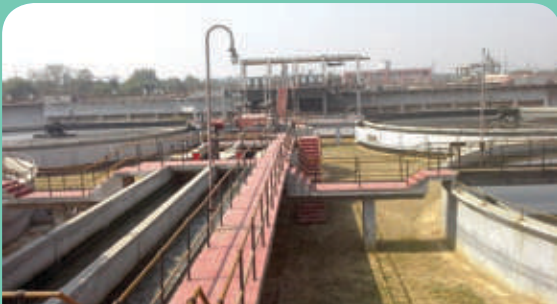
91 MLD Wastewater Treatment Plant Pappankalan, New Delhi, India Large WWTP based on total resource recovery (Arth Ganga)
