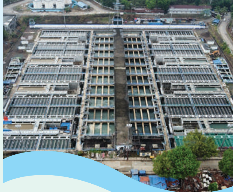
900 MLD WTP, Lamesa, Philippines
