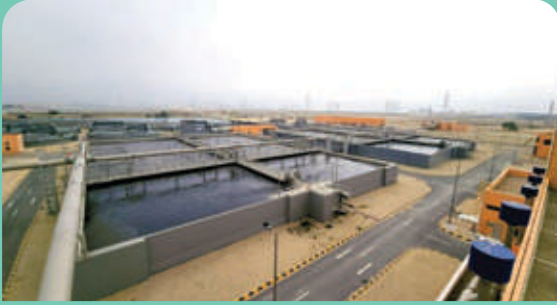
120 MLD Wastewater Treatment Plant (WWTP) Jubail, Kingdom of Saudi Arabia One of the largest wastewater infrastructure in Kingdom of Saudi Arabia
