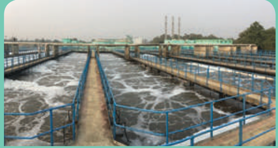
140 MLD Sewage Treatment Plant Dinapur, Varanasi, India First and largest STP inaugurated under 'Clean Ganga' mission
