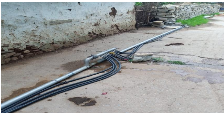
Laying of Water pipeline at Payeri village at Karunda.
