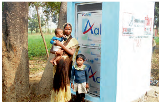
➤ Ms. Asha with her children in front of her newly constructed toilet in village Sarhara, Hallia Block, Mirzapur district, Uttar Pradesh
