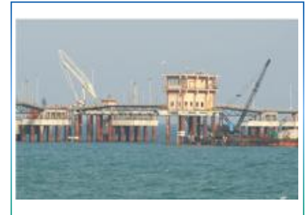
Marine Terminal Facility, Cuddalore, Tamilnadu
