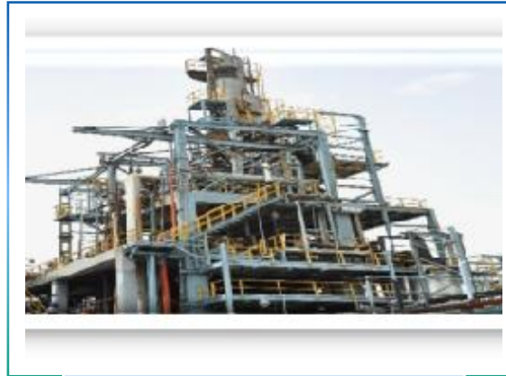
Chloromethanes plant, Mettur, Tamilnadu
