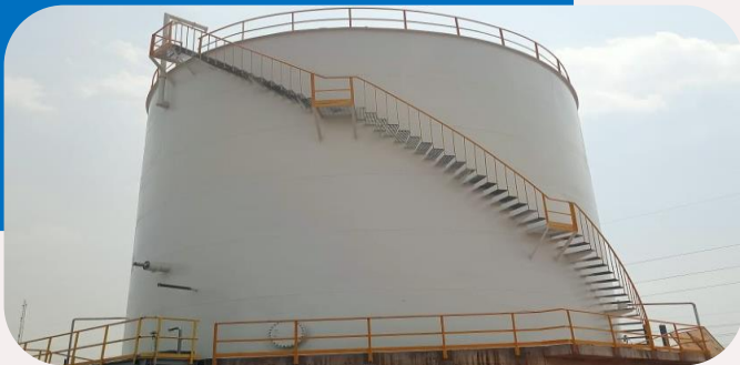
LOX Flat Bottom Tank 900 M3 order received from North India
