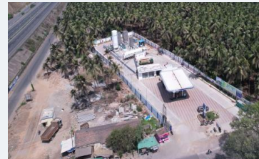
LNG/LCNG fuel stations
