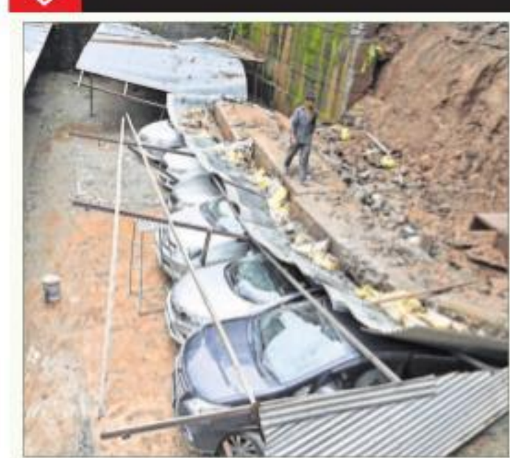
Vehicles crushed under a collapsed wall at a parking place, following rains, in Mandi, on Friday PTI
