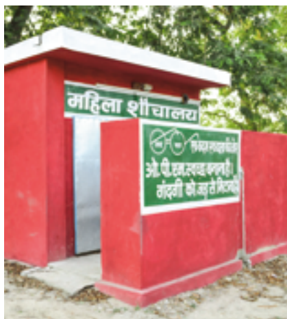
Construction of Ladies toilet
