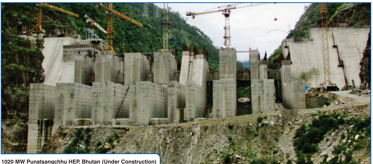
1020 MW Punatsangchu HEP, Bhutan (Under Construction)
