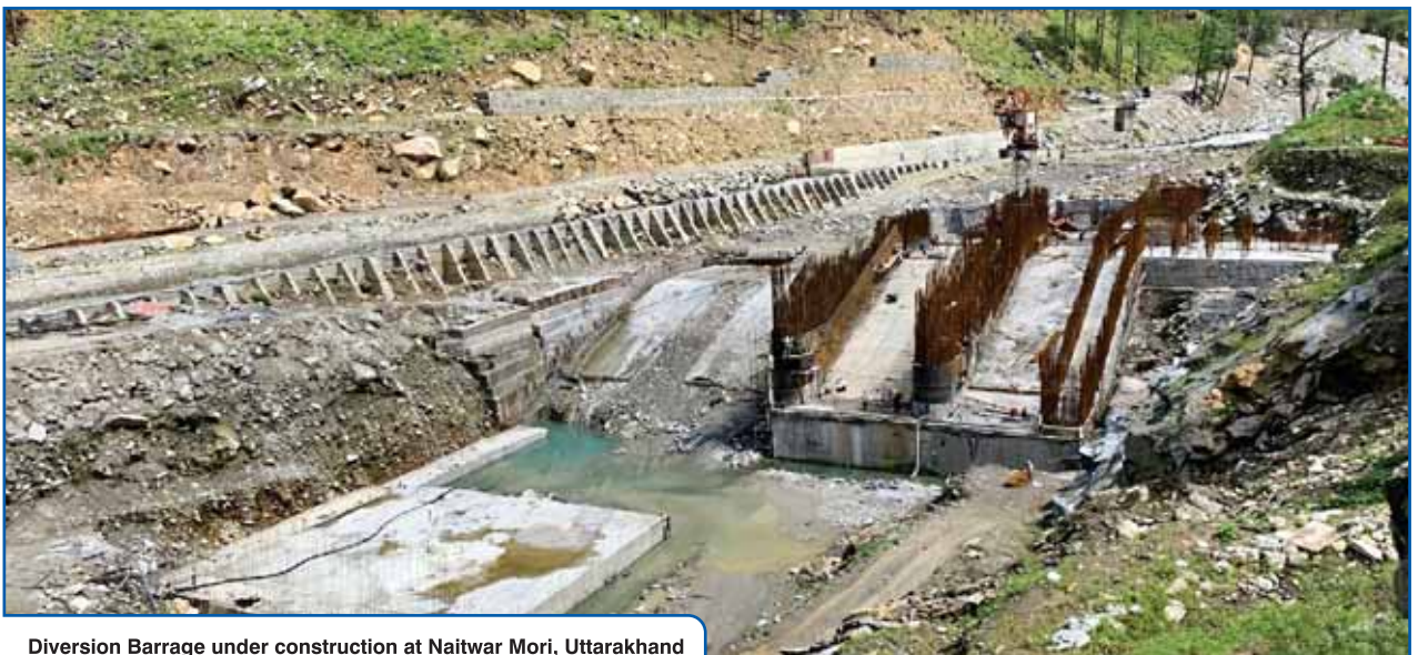
Diversion Barrage under construction at Naitwar Mori, Uttarakhand
