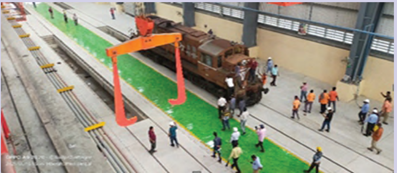
Commissioning of Phase-I Works of the Jheel Siding Coaching Depot at Howrah
