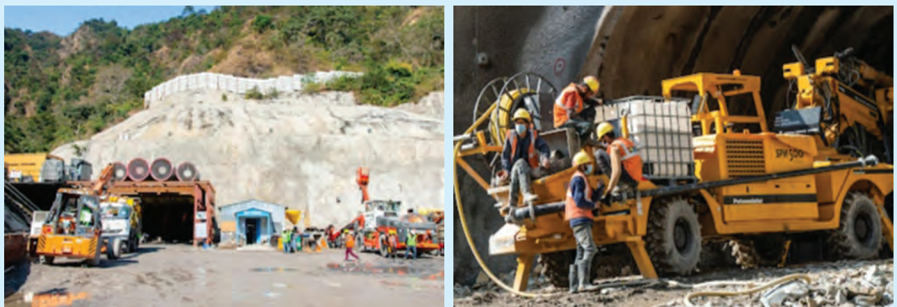
Persevering Team of RVNL marks a landmark achievement through 37 Km Tunneling in the complex geology of Rishikesh- Karanprayag Project
