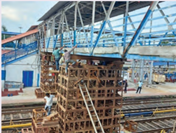
Raising of FOB Over 3 Tracks And 2 Platforms at New Bongaigaon
