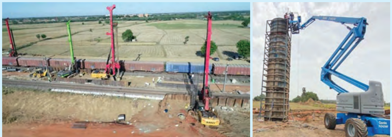
Completion of 525 Piles in Five Months Contiguous to the High-Density Rail Network Near Gudur In Connection with a Rail Flyover Despite Covid Challenges
