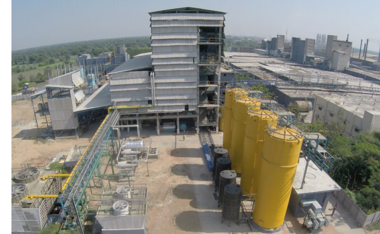
Multiple Effect Evaporator Plant (MEEP)
