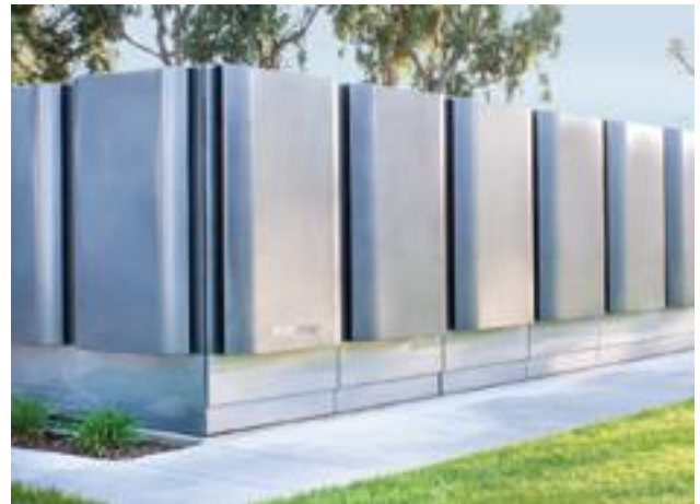
SOFC and Hydrogen units for fuel cells of Bloom Energy
