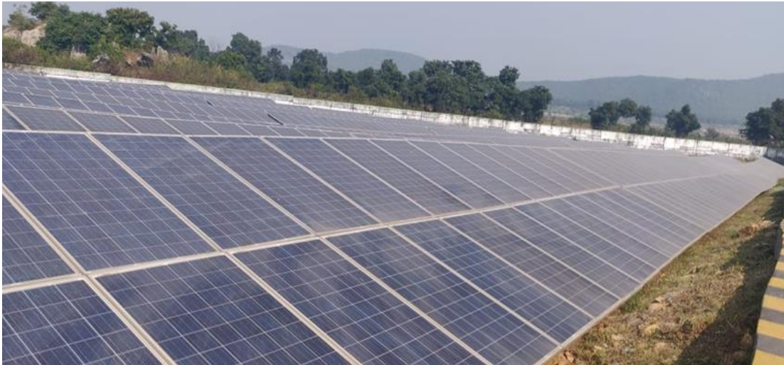
Fig. 67 - Ground mounted Solar Power Project of MCL
