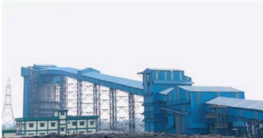
Fig. 36 - Silo in Lingaraj OCP of MCL
