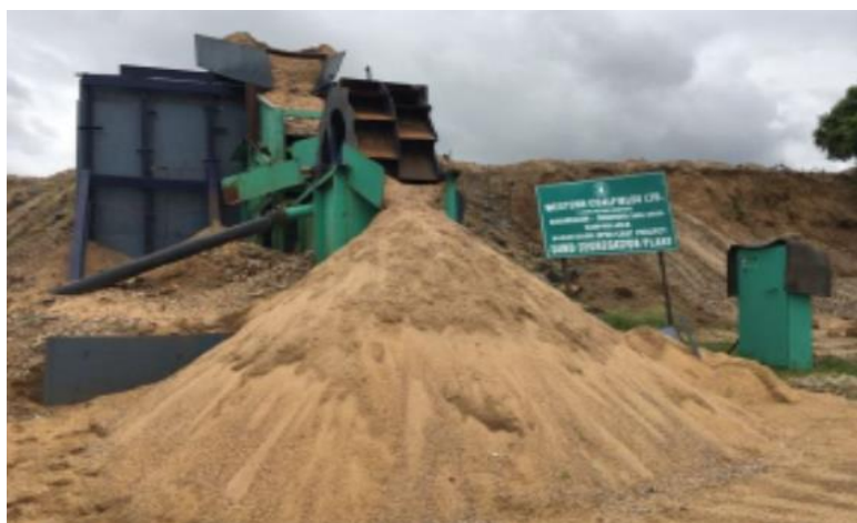
Fig. 65 - Pilot Project of Sand segregation (250 cu.m/day) in WCL
