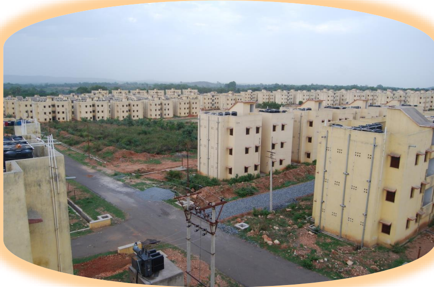
Fig. 26 - Rehabilitation site in BCCL
