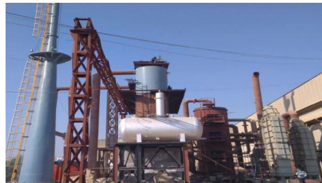
Kisan Phosphates, Haryana: Fertilisers Plant
