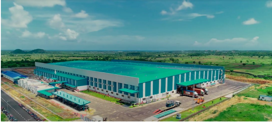
TCPL's largest tea packing plant set up at Gopalpur Industrial Park
