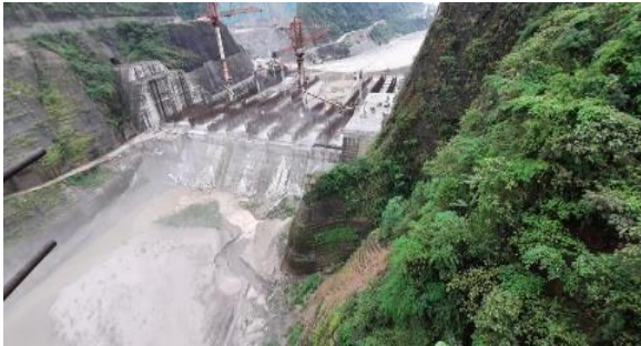
Subansiri HE Project 2000 MW project in Arunachal Pradesh
