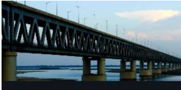
Bogibeel Bridge, Assam The largest Rail and Road Bridge in India
