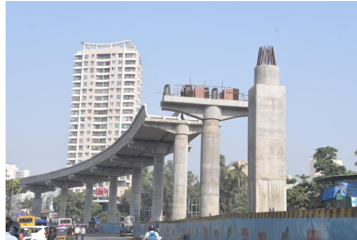
Mumbai Metro Line 9
