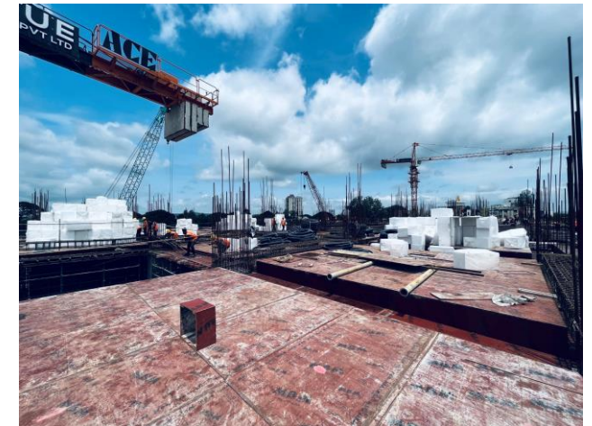
Pune Underground Metro
