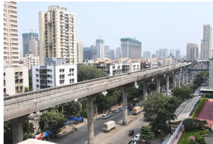
Mumbai Metro Line 6
