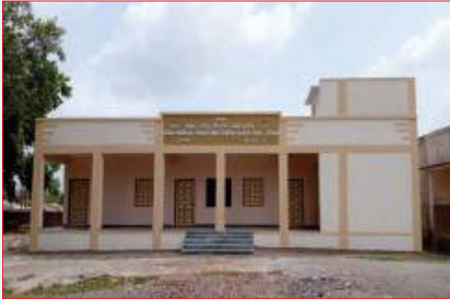
Construction of Class Room, Bodhan
