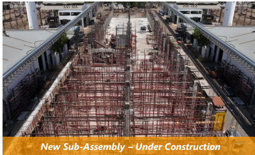
New Sub-Assembly – Under Construction
