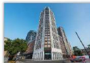
Apex House Location: London, UK Supplier: Vision Modular Systems UK
