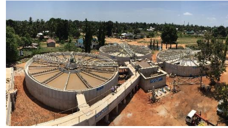
130 MLD Drinking Water Treatment Plant, Tanzania First water project in Africa to be commissioned under EXIM India funding
