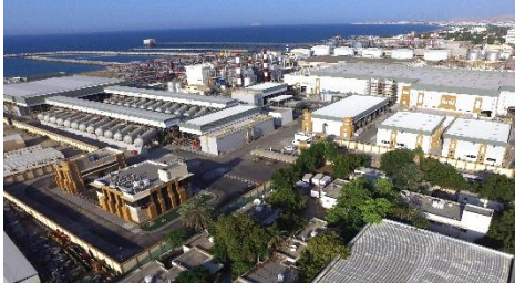
191 MLD SWRO (Desalination) Plant, Al Gubrah, Oman Largest desalination plant in the country of Oman
