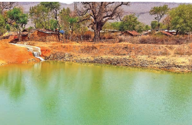
Water harvesting at Barghar Mines
