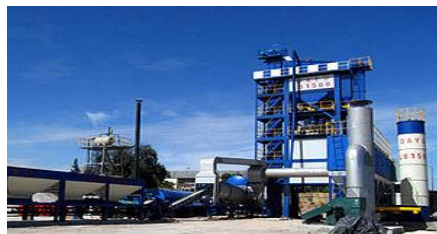
Contractor Camp Mobilization
