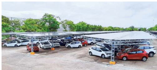
The 6.2 MWp solar carport will generate 86.4 lakh kWh of electricity per year and is estimated to reduce 7,000 tonnes of carbon emissions annually and 1.6 lakh tonnes over its lifecycle
