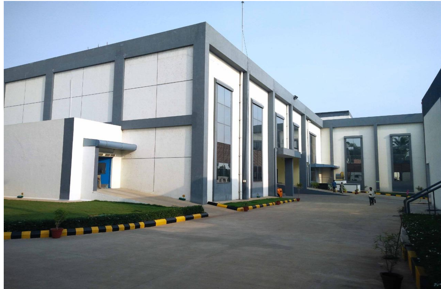
CP-I plant at Suthukeny, Puducherry
