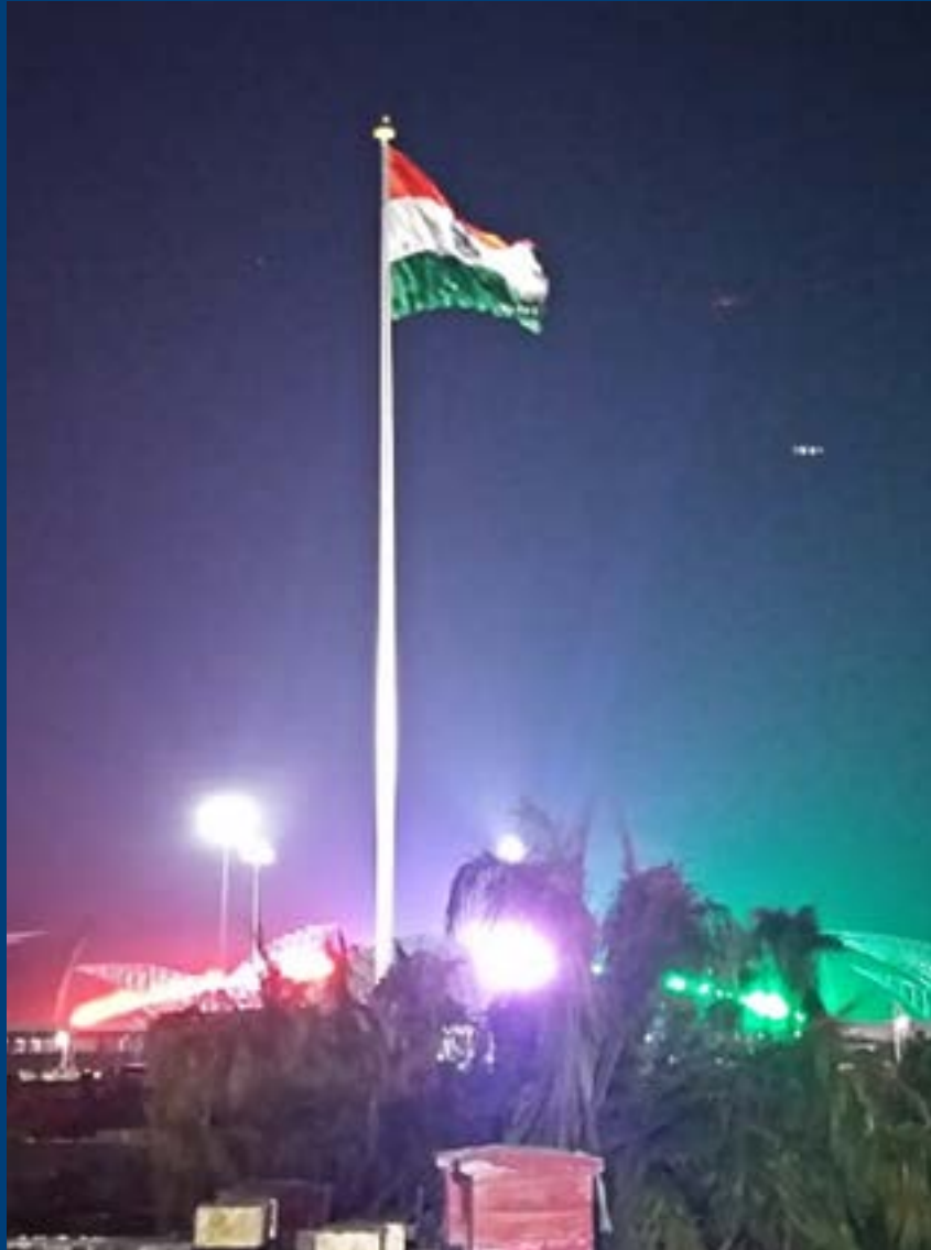
Skipper erected one of the tallest Flag Masts of India, a 300 feet National Flag Mast with 3 nos. of 20m High Masts in Kartarpur Sahib Corridor, Punjab.
