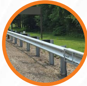
Metal Beam Crash Barrier
