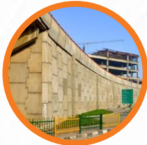
Reinforced Earth Walls
