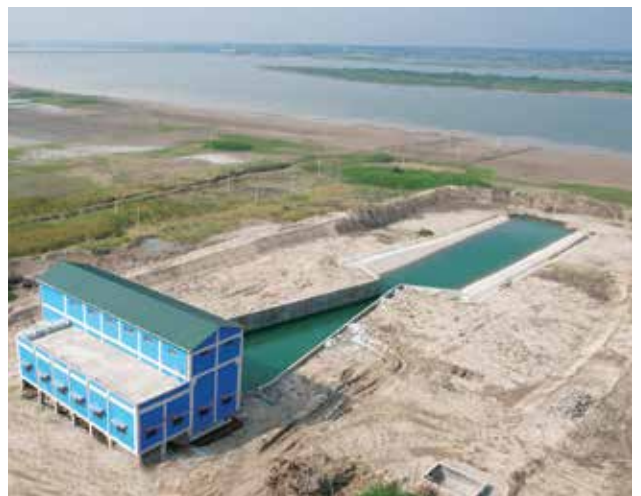
Jack Well Cum Pump House for Minor Irrigation and Ground Water Development Division, Koppal Kushtagi, in Karnataka
