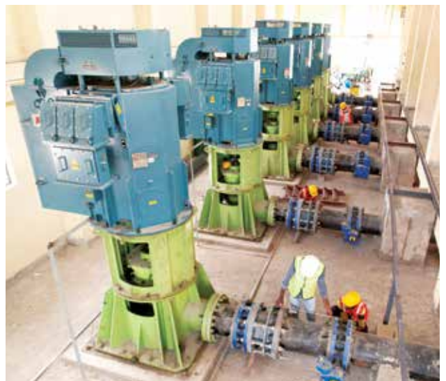
Installation of Pumping Machines at for Minor Irrigation and Ground Water Development Division, Koppal Kushtagi, in Karnataka
