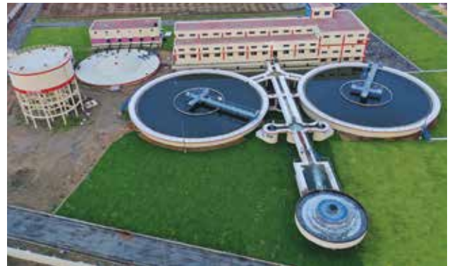
25.51 MLD Water Treatment Plant at Pallakapalayam in Alampalayam Combined Water Supply Scheme for Namakkal & Salem Dist, in Tamilnadu.
