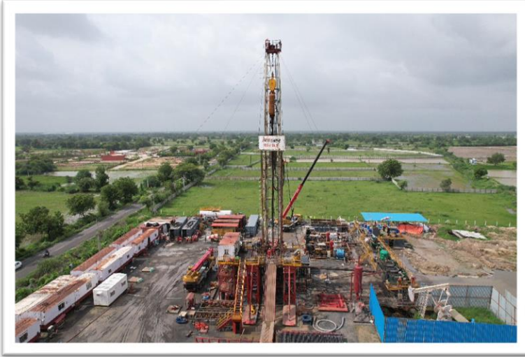
Drilling in Karjisan
