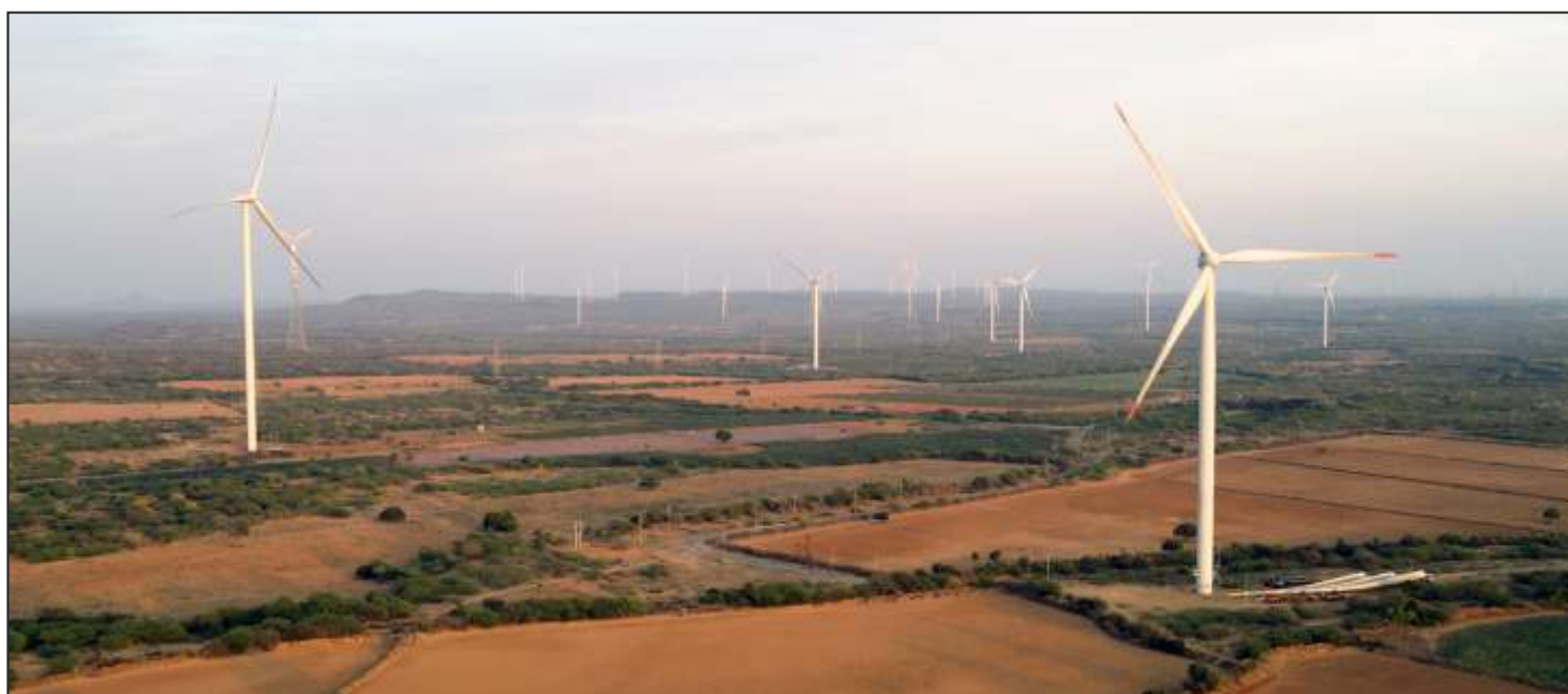
IREDA funded 300 MW Capacity Wind Power Project of M/s Netra Wind Private Limited located at Kutch District, Gujarat.
