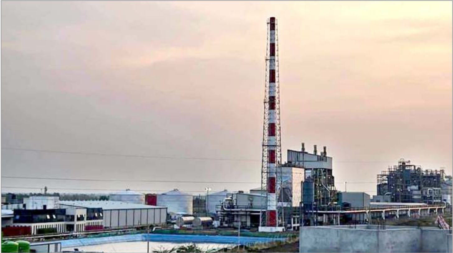
IREDA funded 300 KLPD Ethanol Project of M/s Greenergy Bio Refineries Pvt. Ltd. located at Ranebennur Taluk Haveri District, Karnataka.
