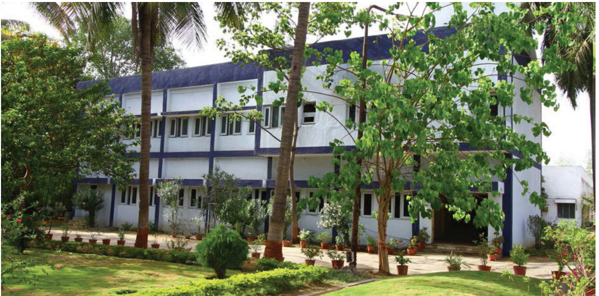
office building at Ankleshwar, Gujarat
