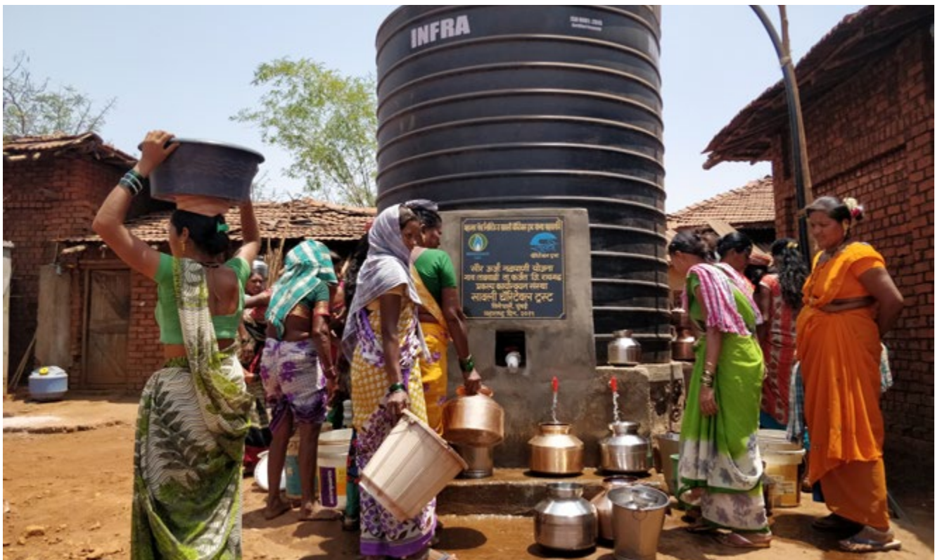
Providing safe drinking water in villages of Karjat
