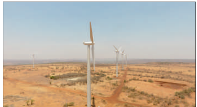
A view of BEML Windmill Project
