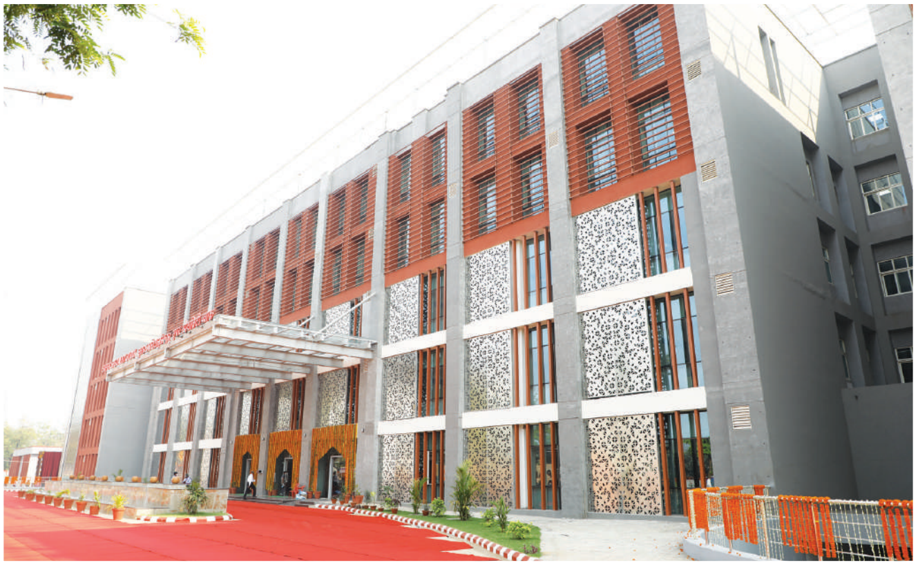
Super Speciality Hospital, Rourkela, Odisha
