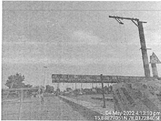
Pullur Toll Plaza
