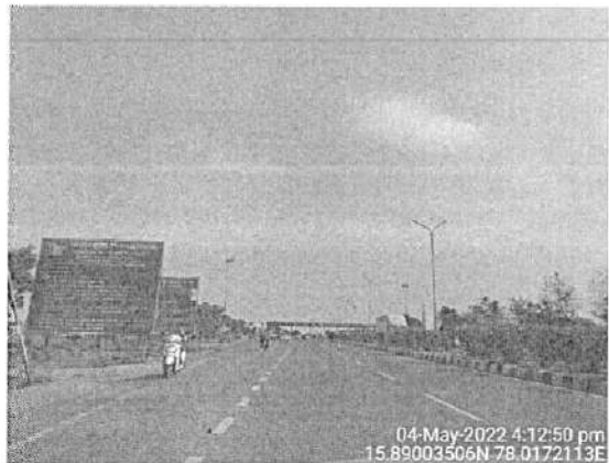
Pullur Toll Plaza
