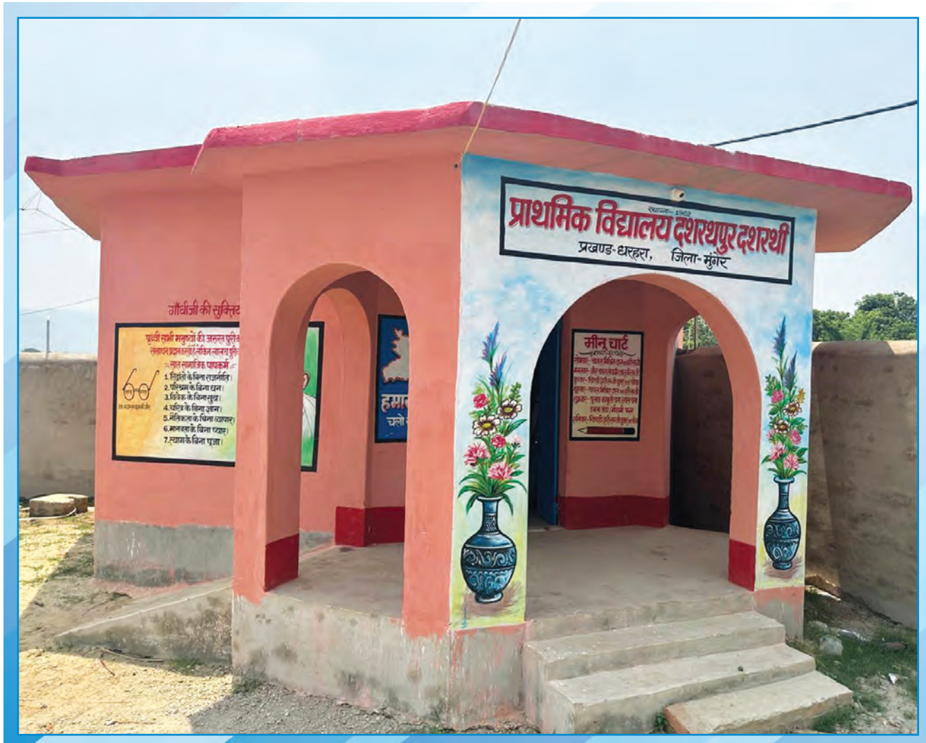
Renovation works at Govt. School, Munger
