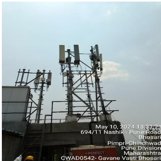
Vitthal Arcade, Bhosari, Pune
