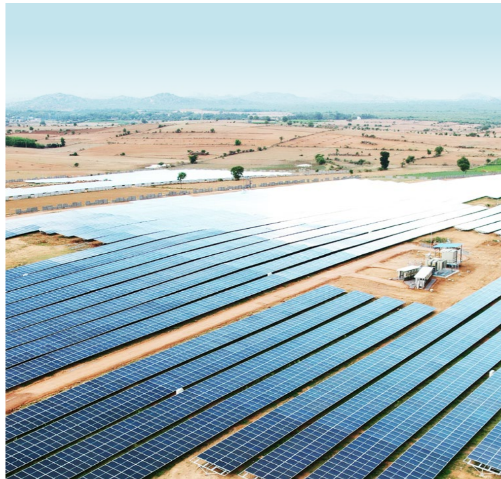
Actual site photo of the 42.9 MW renewable energy project
