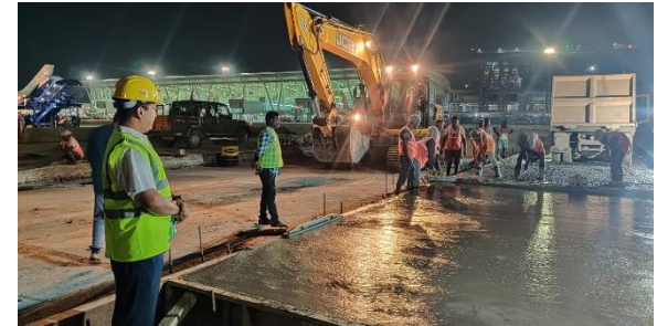
International Airport Taxiway Project, Chennai
