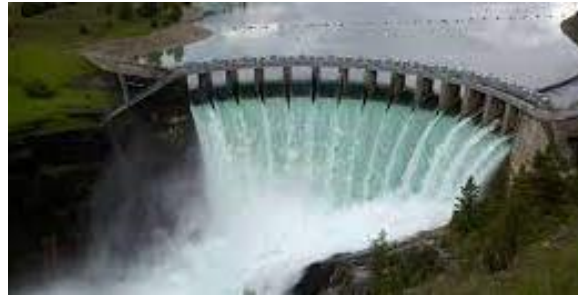
Kopili Hydro Electric Project, Assam
