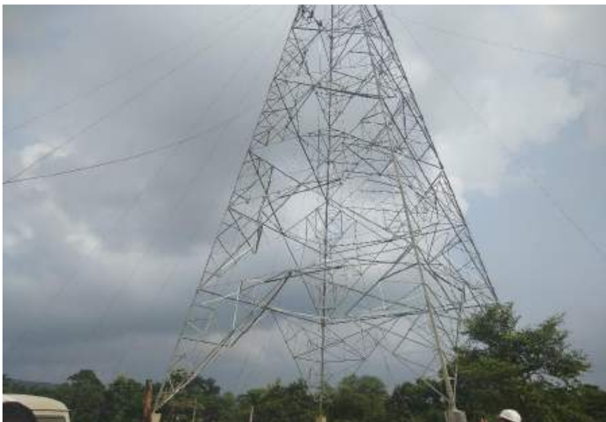
Location 108/3 – Tower erection in progress
