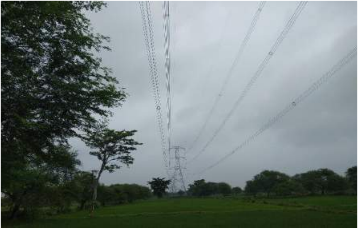
Stretch 1/0 to 4/0 – Stringing complete
