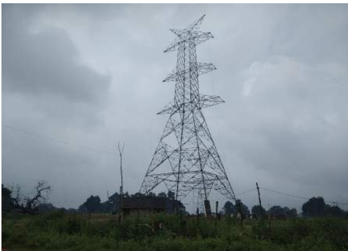
108/4 to 108A/0 – Tower erection complete
