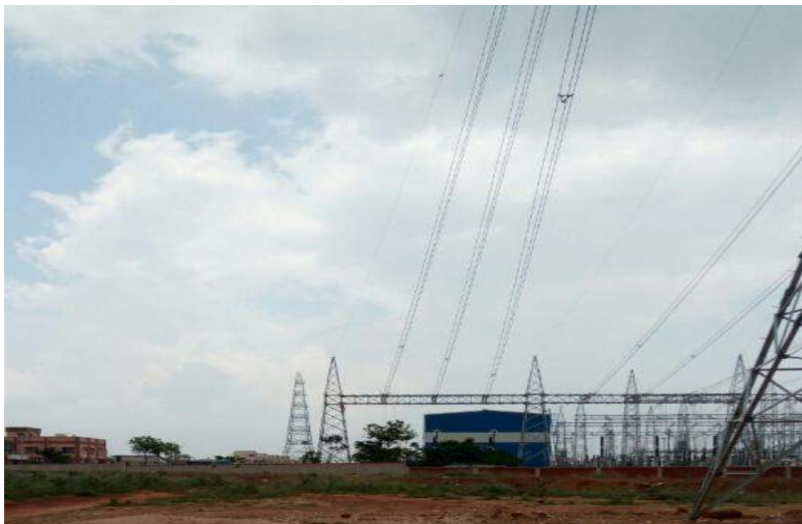
Sundergarh PGCIL substation – Gantry connection complete
