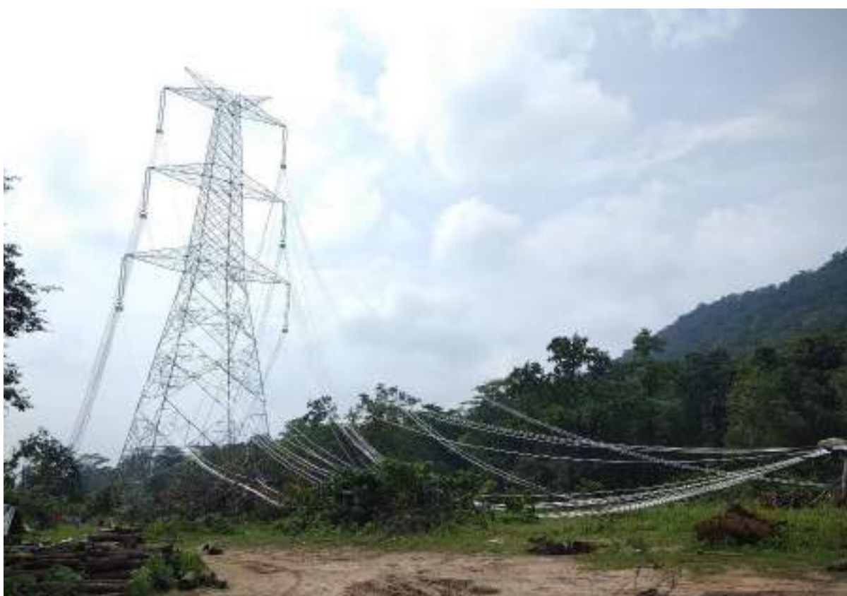
Stretch 115/6 to 116A/0 – Stringing in progress
