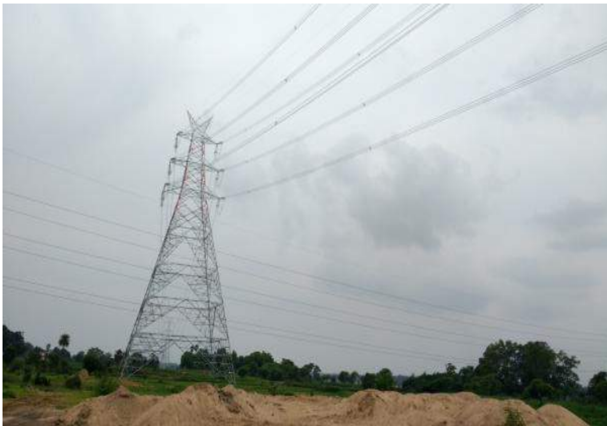
Stretch 32/0 to 33/0 – Stringing complete
