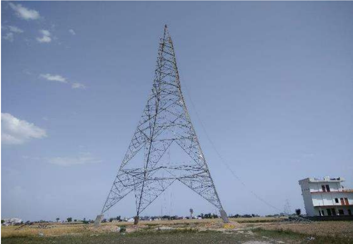
Location 34/0 – Tower erection in progress
