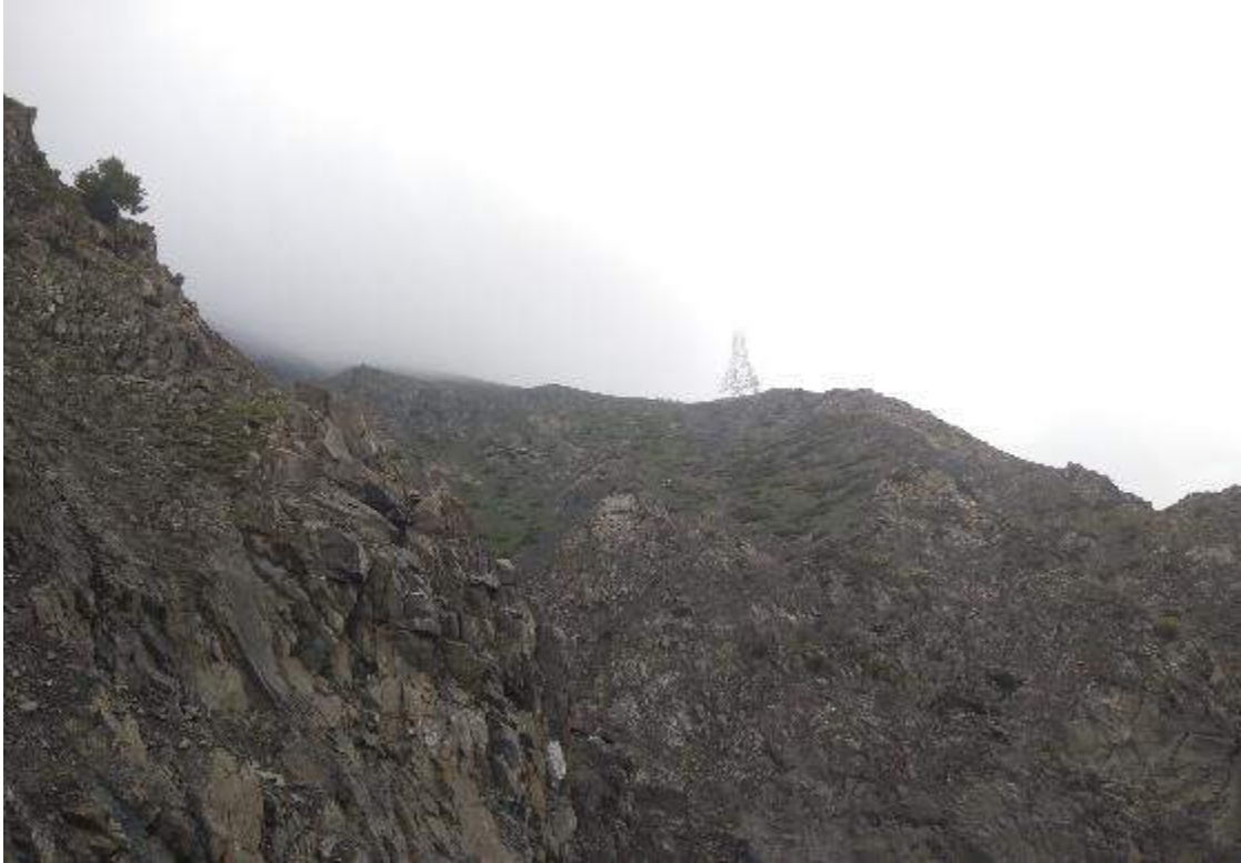
Location 338/1 – Tower Erection in progress
