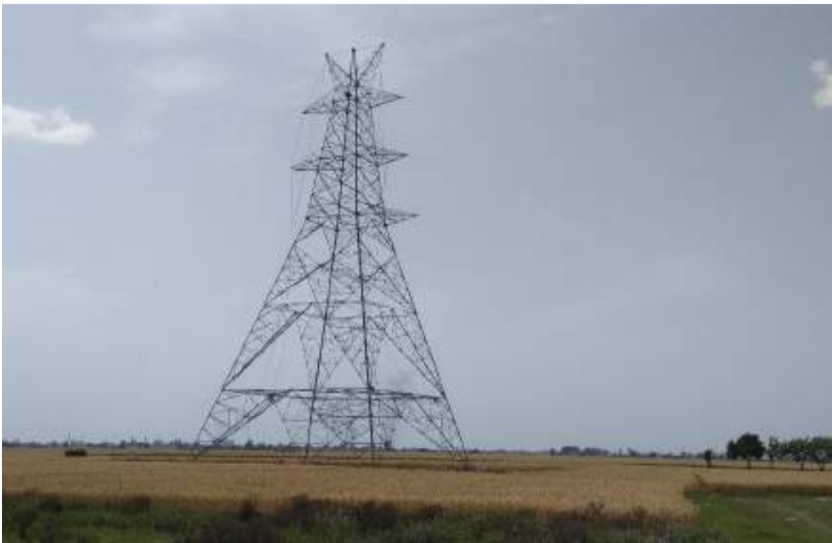
Location 35/0 – Tower erection progress
