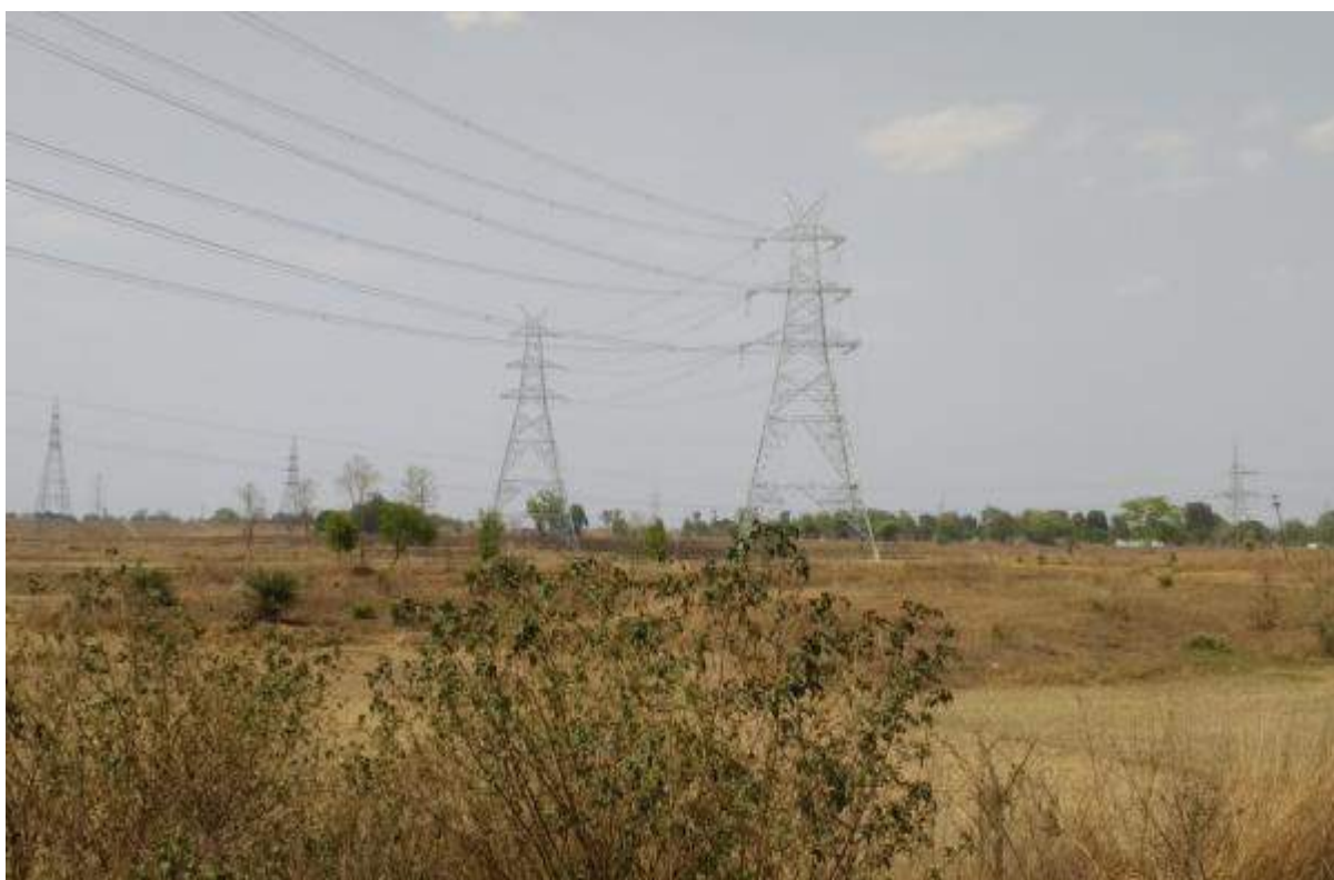
Stretch 30/0(DD+18) to 35/0 (DC+0) – stringing complete
