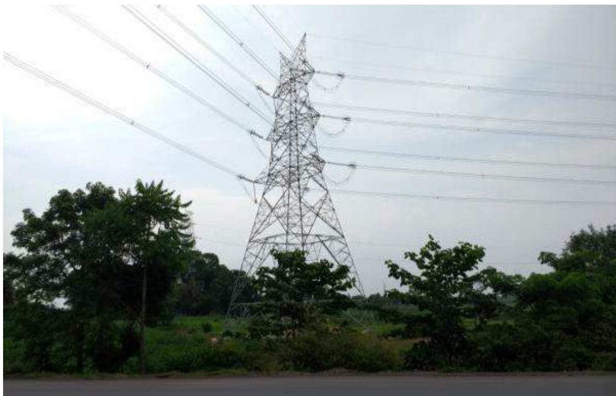
Location 32/0 – Road crossing, Erection and stringing complete
