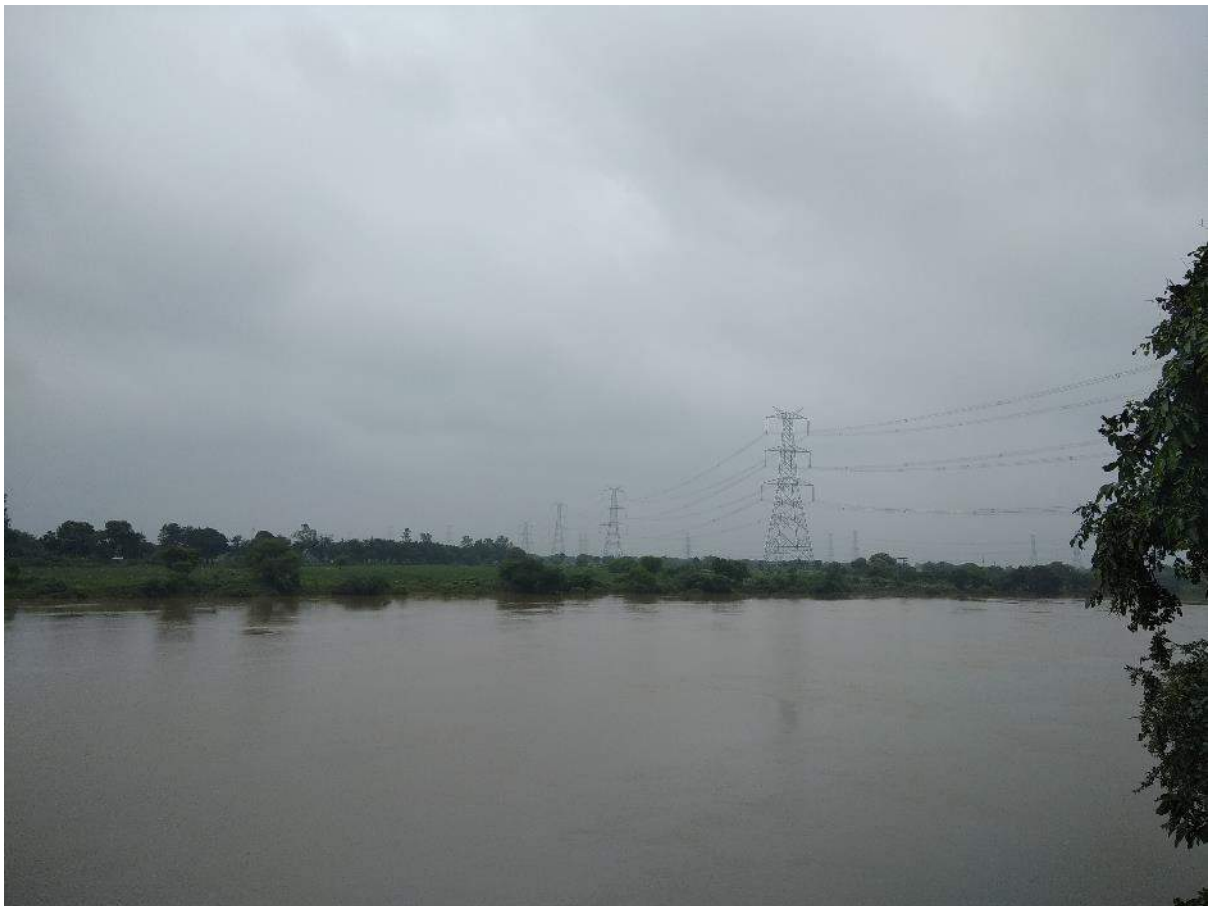
Section 2/3 & 3/0 – river crossing stringing complete
