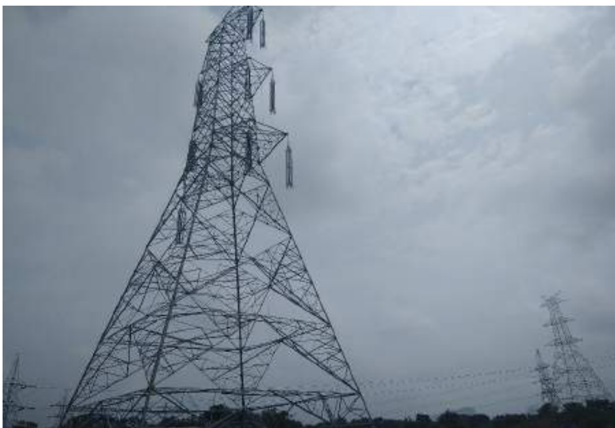
Section 105/0 & 106/0 – Stringing works to start
