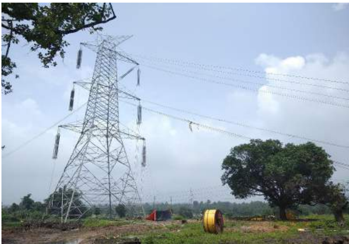
Location 115/0 – Stringing works are in progress
