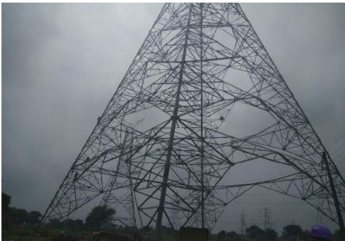
Location 104A/0 – Tower erection in progress
