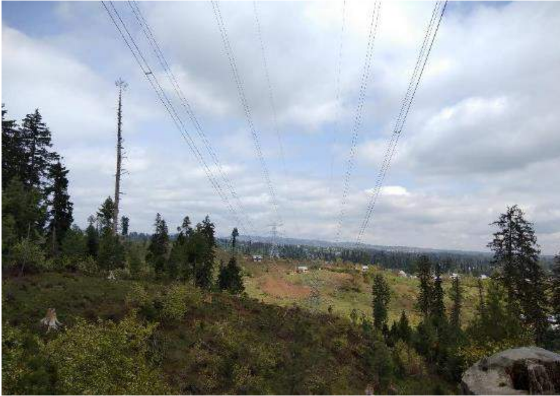
Stretch 409 to 413 – Stringing along with OPGW is complete
