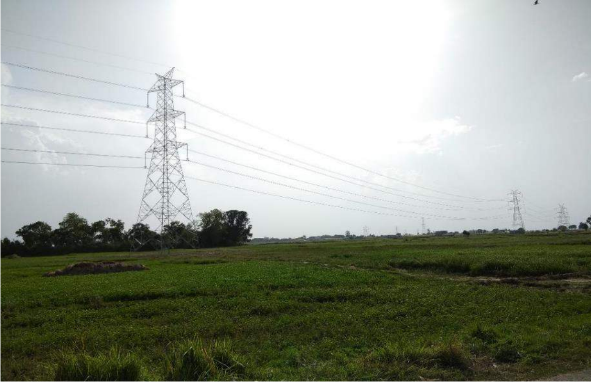
Stretch 20/3 to 30/9 – Stringing complete
