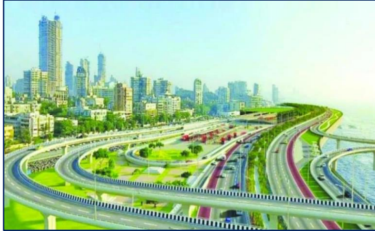
MUMBAI COASTAL ROAD (MUMBAI, MH)
