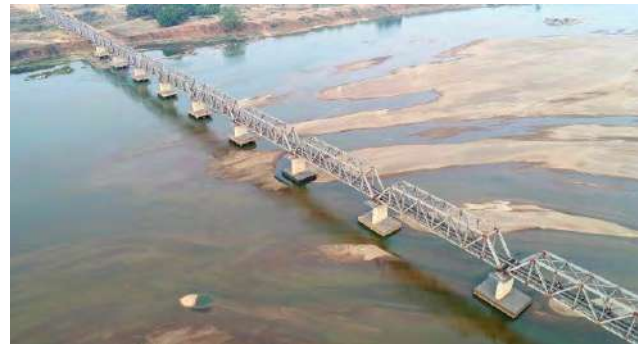
Bridge no. 12 on river Brahmani
