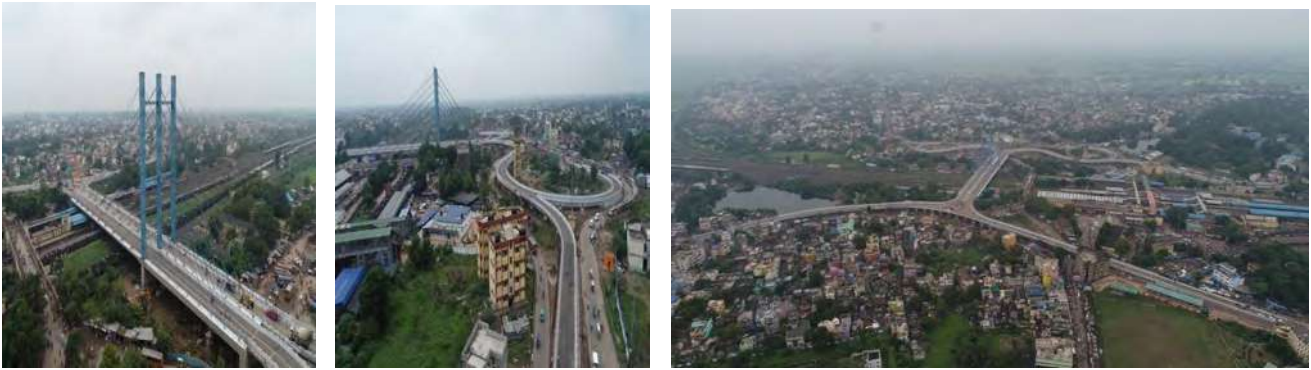
4-lane Cable Stayed Bridge over busy Barddhaman Yard along with its 3.5 Kms long approaches commissioned in Sep 2019.
