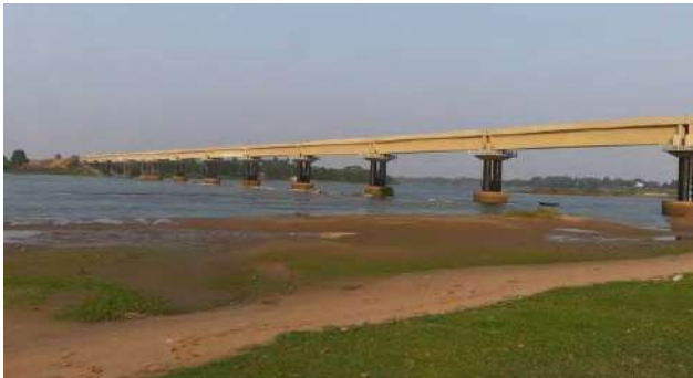
Bridge no. 134 over River Mahanadi
