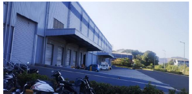
Building No B200, Shed 200, Indran Logi Indospace Industrial & Logistics, Ajivali, Khalapur Raigad - Khopoli
