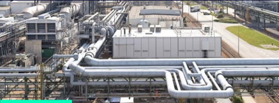
Electrification, Automation & Digitalization solutions
