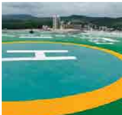
Leading Hotel Helipad work completed with Luxurea MP 500 and Pro Polyshield UV 75.
