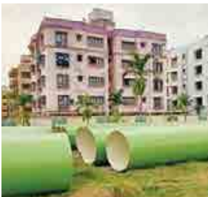
Bergerthane Solvent Free HB coating was successfully applied on drinking water pipeline project under PHED Kolkata, and Kolkata Environmental Improvement Project.
