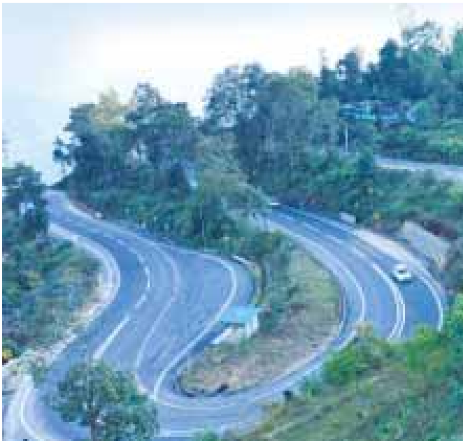
Thermoplastic Road Marking (Sigmark) at Rehnok-Pakyong Road Project- Sikkim (National Highway- 717A)
